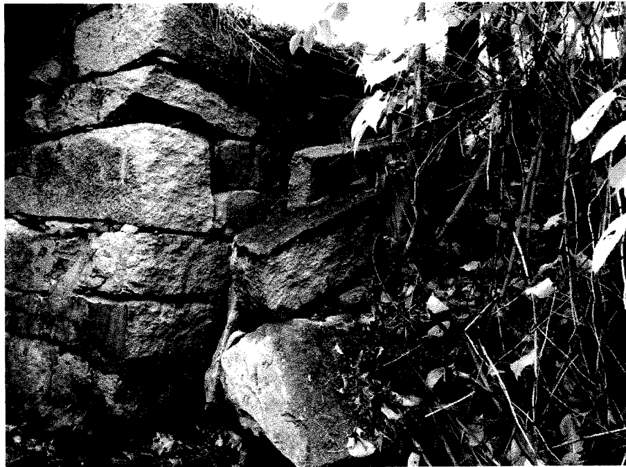
PHOTO 8 Description NE retaining wall
