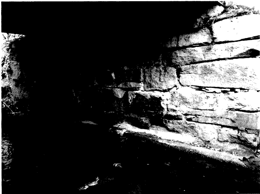
PHOTO 7 Description North abutment
